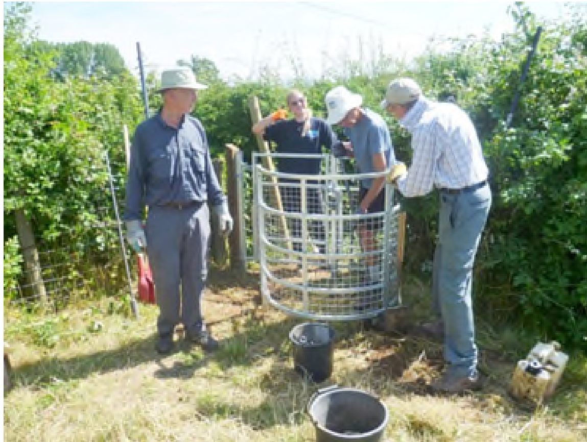
Installing a kissing gate
